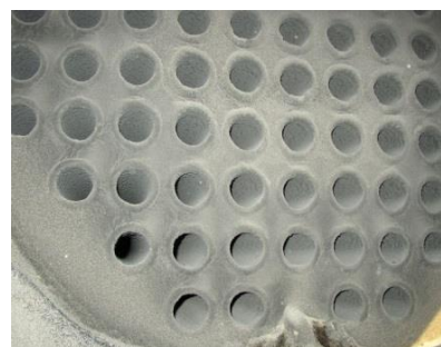
Figure 4-19: Fire-tube boiler (opened) [74]
